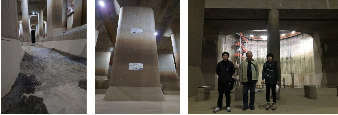
Sediment in the corner of the tank / Small-sized pillar (upper and lower limits of the water level) / At the connection with the first shaft (Inaba, Yamamura, Miwada)
