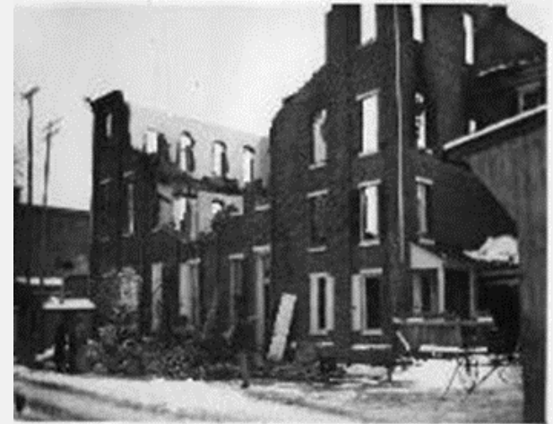
Kerosene Lamp on Stage Knocked Over Igniting Combustibles.
