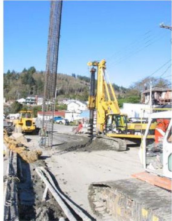
Photo 2. Shear Pile Remediation of a Landslide on the Oregon Coast
