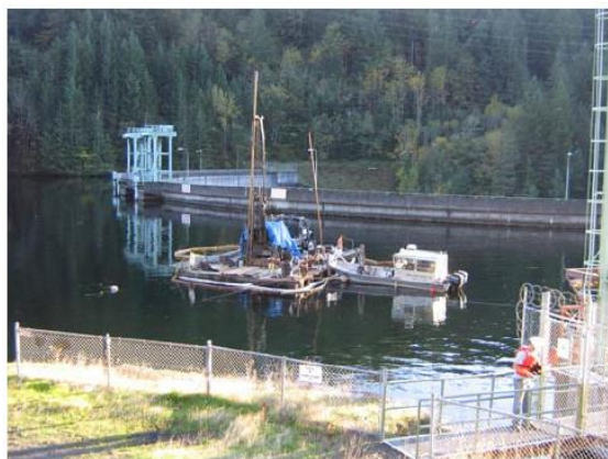
Photo 1. Overwater Drilling Behind a Concrete Arch Dam
