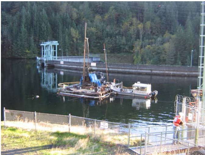
Photo 1. Overwater Drilling Behind a Concrete Arch Dam
