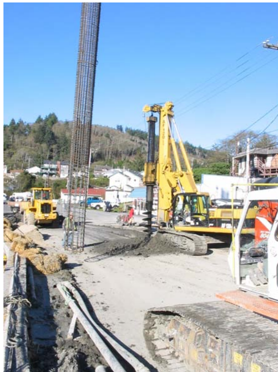
Photo 2. Shear Pile Remediation of a Landslide on the Oregon Coast
